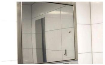
Professionally installed Mirror Shield restores the surface and protects it from future vandalism incidents including paint, scratches, markings and even acid etching. The application and/or replacement process is quick ensuring minimal impact on daily business and operations.
