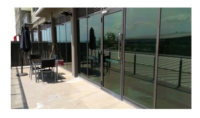
Temperature logging of the suites, one with film applied, the other without, revealed a large difference in interior room temperatures during the sunniest times of the day
